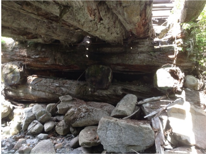
Right Bank Abutment when facing downstream
