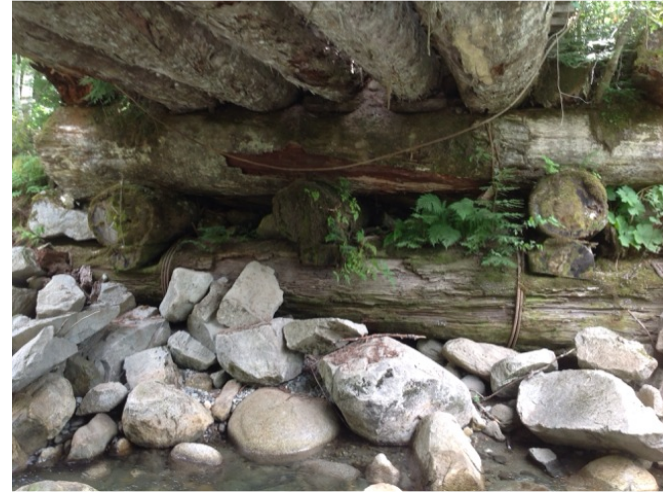
Left Bank Abutment when facing downstream
